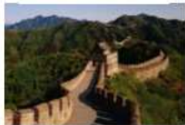
The Great Wall of China
